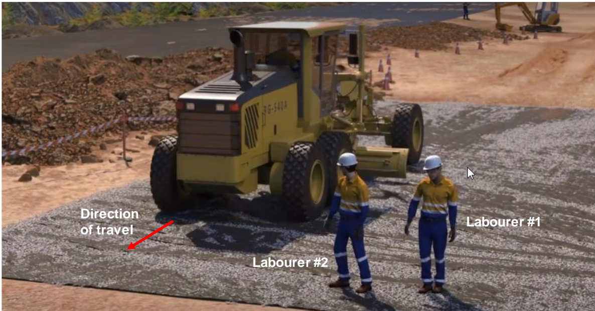
Fig. 4: Location of the grader and Labourers at the time when the Labourers observed the grader reversing in the close proximity to them.
