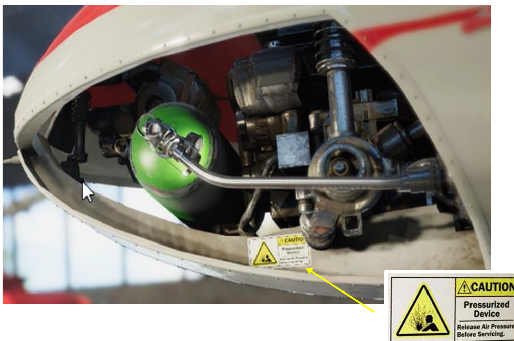
Fig. 4: Placard warning and its location in nose section of the helicopter.
